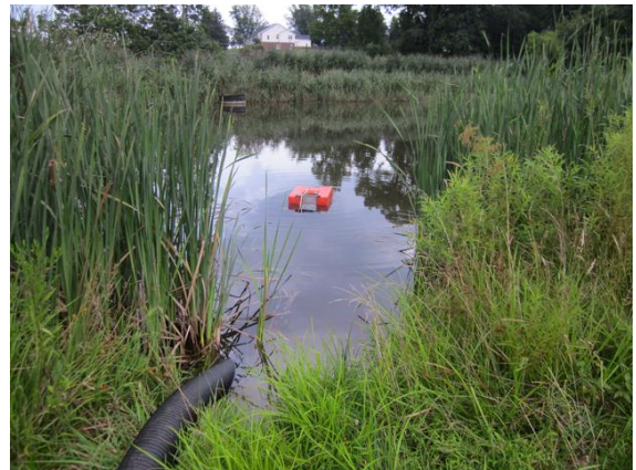
Test #2 - a floating suction strainer was used in lieu of the dry fire hydrant because of an air leak in the head.
