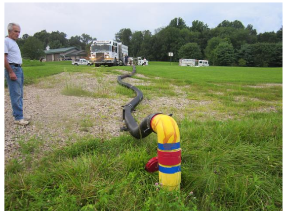
In addition to the 100 feet of suction hose, the dry fire hydrant added about another 10 feet of 6-inch pipe from which air had to be evacuated.
