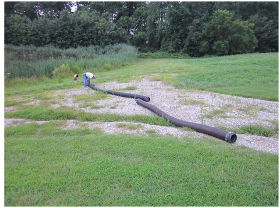
Members work to lay out and connect the 100 feet of suction hose.
